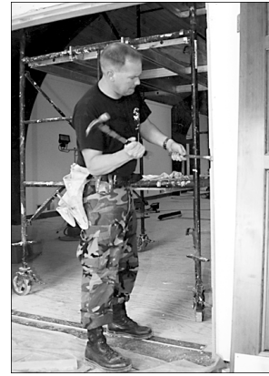
LEFT: Senior Airman Bill Christopher repairs a door frame as part of renovations in the Annex Assembly Hall.
